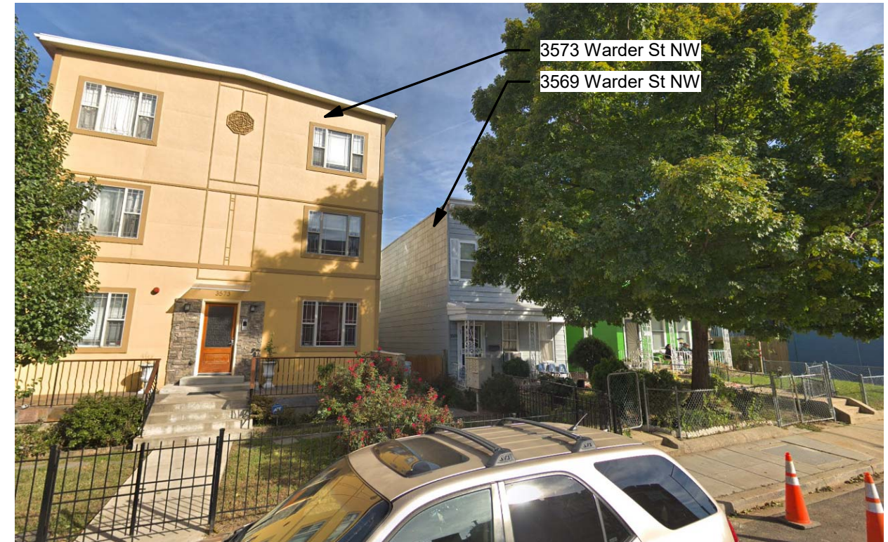
FROM STREET (SHOWING 3573 WARDER ST NW)
